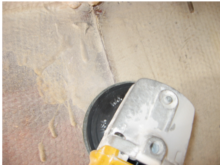
Figure 3 Side grinder with 60 grit for removal of old tabbing
