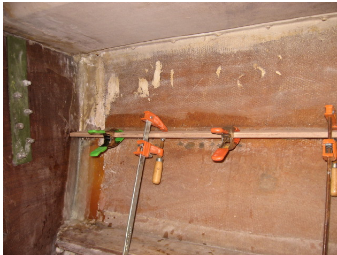
Figure 26 New shelf clamped onto old tabbing
