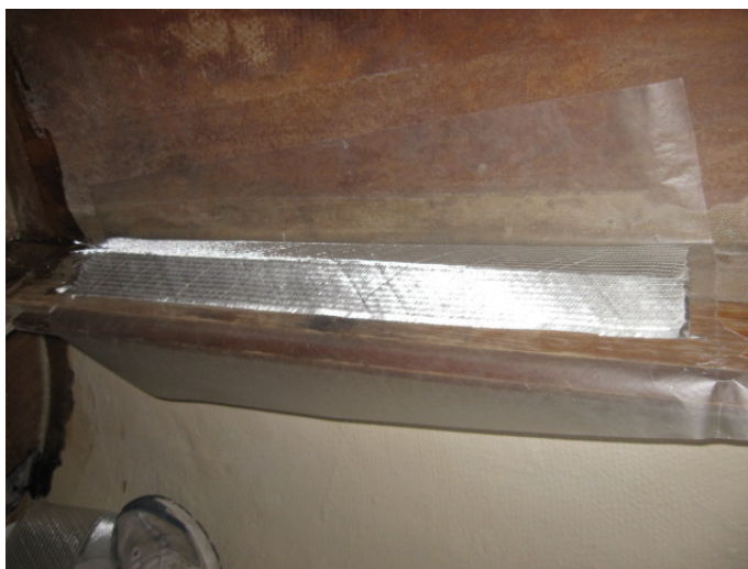
Figure 18 Tabbing tape pre-creased for corner
