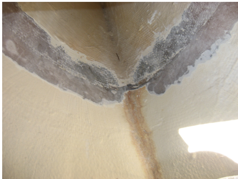
Figure 5 Tabbing ground out and area smoothed
