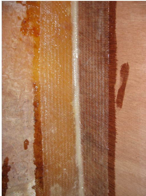
Figure 20 Close up of finished filleted tabbing
